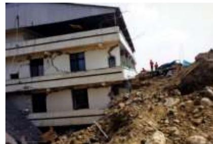
Fig. 1. Damages of building caused by reverse faulting in the 1999 Chi-Chi earthquake (Provided by W.J. Huang, NCU)
